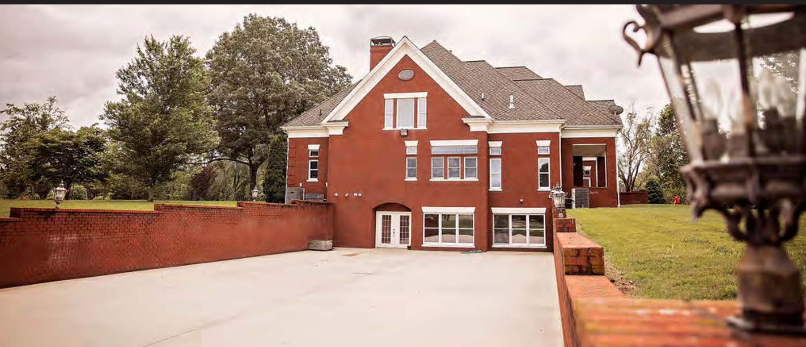
North side of home with parking area and separate entrance to the basement level
